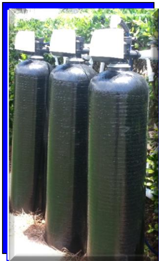
The Iron Eliminator Treats Up to 100 ppm of iron in water.
